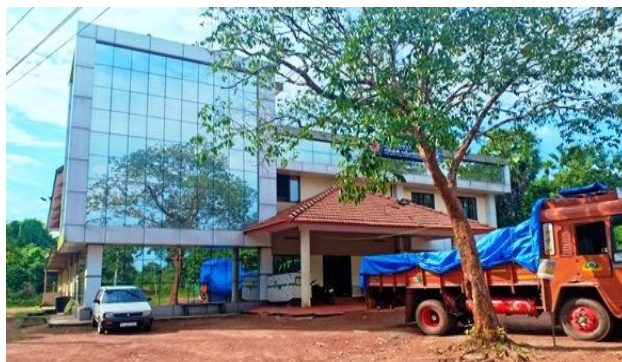
Figure 2.1: Civil Defence Training Institute Building 29 October 2019, CDTI, Viyyur, Thrissur District Photo taken by Audit party, attested by Director, Fire and Rescue Services Academy
